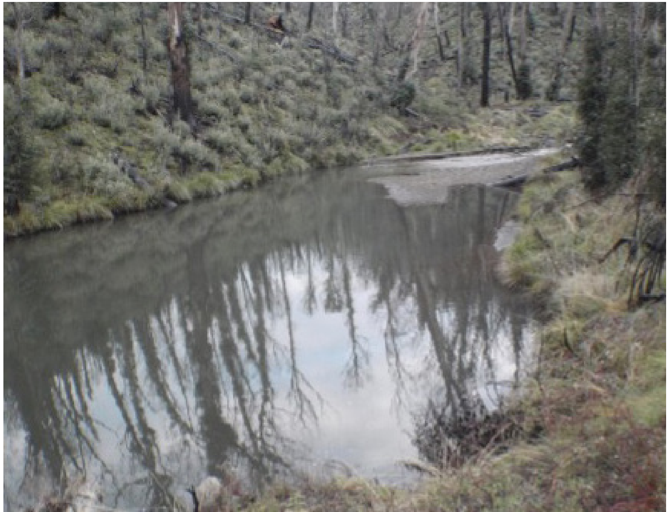
Rules Creek Dam with silt - Yarrangobilly's water and hydro power source. The rain event, after the fire, when the hills had little vegetation cover deposited large amounts of silt into the waterways and dam. This limited the capacity of the hydro plant to produce electricity. The dam was unable to be desilted during the winter because the wet ground and steep terrain made it too dangerous for the excavator to access the site. The lack of power limited Yarrangobilly's ability to utilize all show caves by using electricity.
