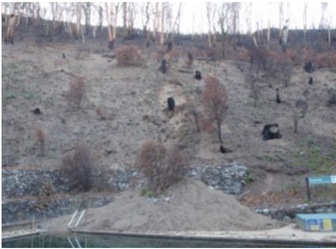
Thermal Pool after the first major rain event. The steep terrain, loose soils and the vegetation denuded slope resulted in soil sliding into the pool. The large Eucalyptus trees which once grew on this slope were removed after damaged sustained in the 2003 fires. Only their stumps remain.
