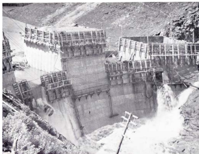
Myponga Dam Under Construction and in Flood September 1960
