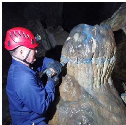
Figure 5 Removing stubborn paint with a mildly abrasive brush attached to a drill.
