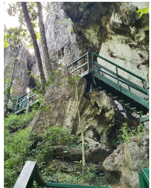
Walkway constructed through the karst leading to the cave entrance (above)
